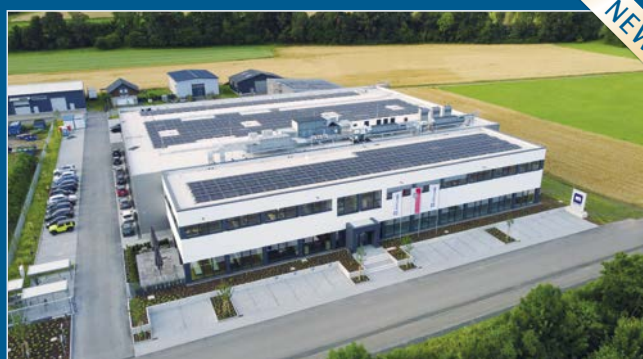
The new building will now expand the current capacity (photo: MULTIVAC)
